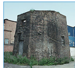
Watsons' Mill prior to any renovation work commencing.
