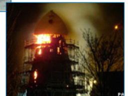
Fire at Watsons' Mill during renovation work in January 2008.
